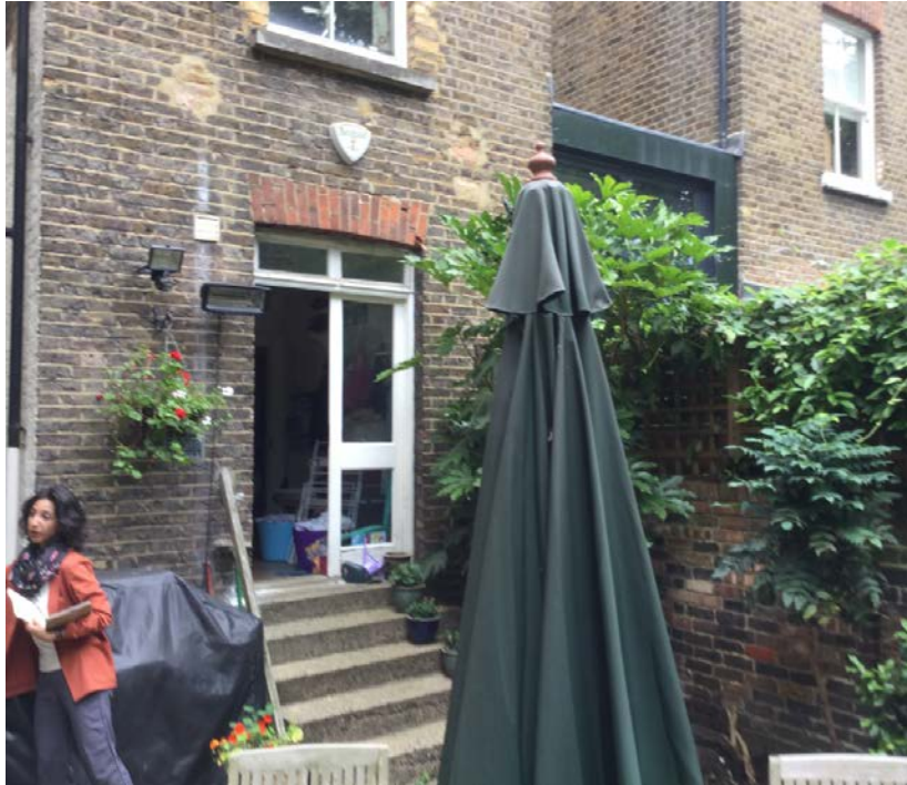
View of location of two storey rear extension to the closet wing at lower ground and ground floor levels.
