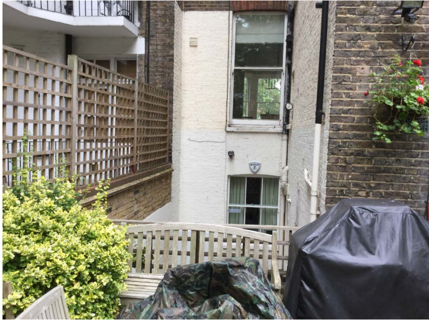
View of location of single storey lower ground floor level infill extension.
