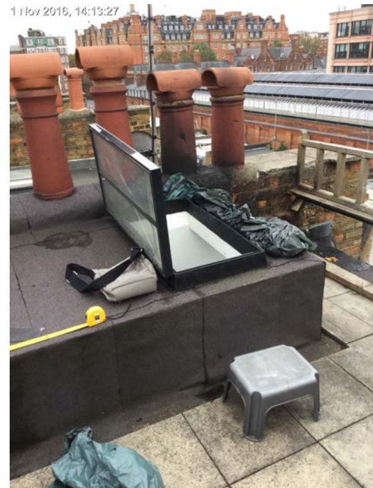
Front elevation (top) and existing access hatch at roof level (bottom).
